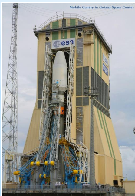
Mobile Gantry in GSC
